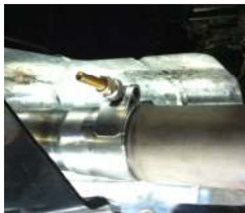
New SPI Clamp Installed
