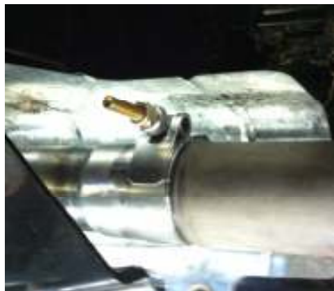
New SPI Clamp Installed
